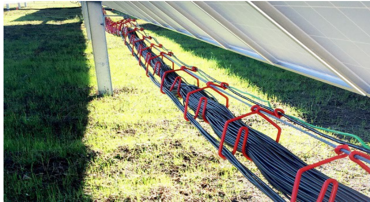
Figure 7. DC Cabling Hanging Harness System
