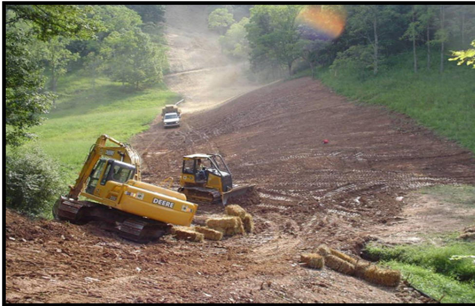
Figure 4.2.9-2 Erosion Control
