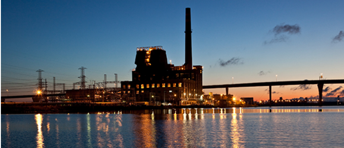
Figure 1: Hibbard Renewable Energy Center
