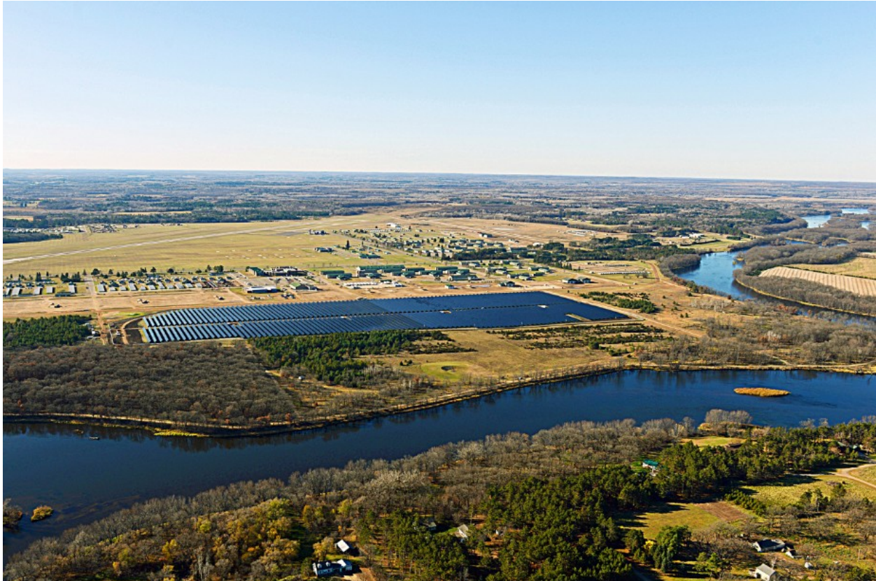
Figure 9: Camp Ripley Solar Project
