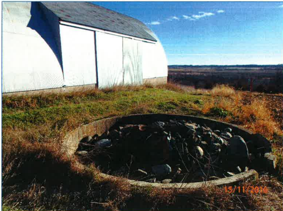
Figure 59. Feature 4 and Feature 7: Silo foundation and metal shed view to the southeast.
