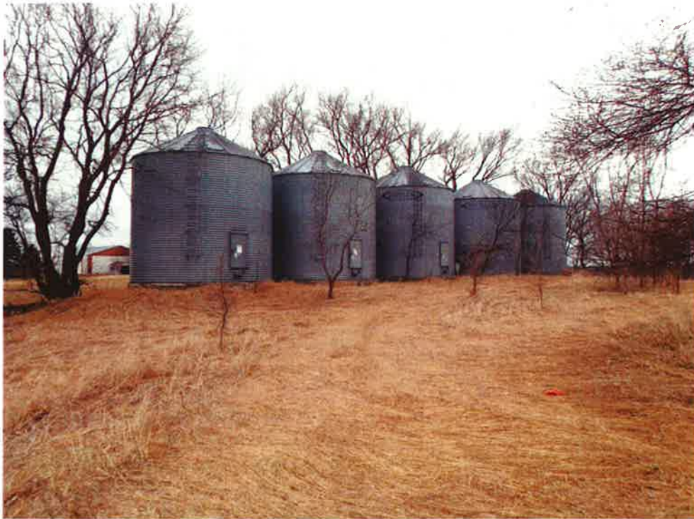
Figure 91. Five modern metal grain silos, looking to the southwest.
