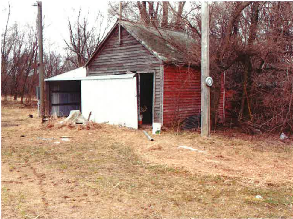
Figure 83. Feature 3, a garage, looking to the southwest.
