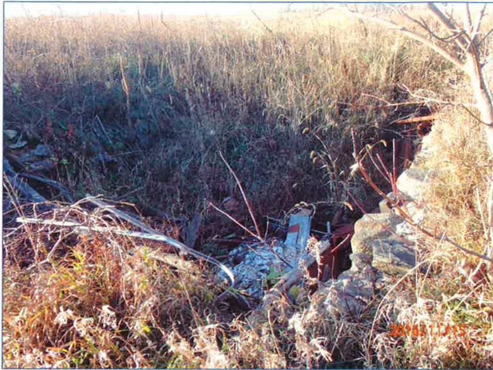
Figure 60. Feature 5: Foundation view to the northwest.
