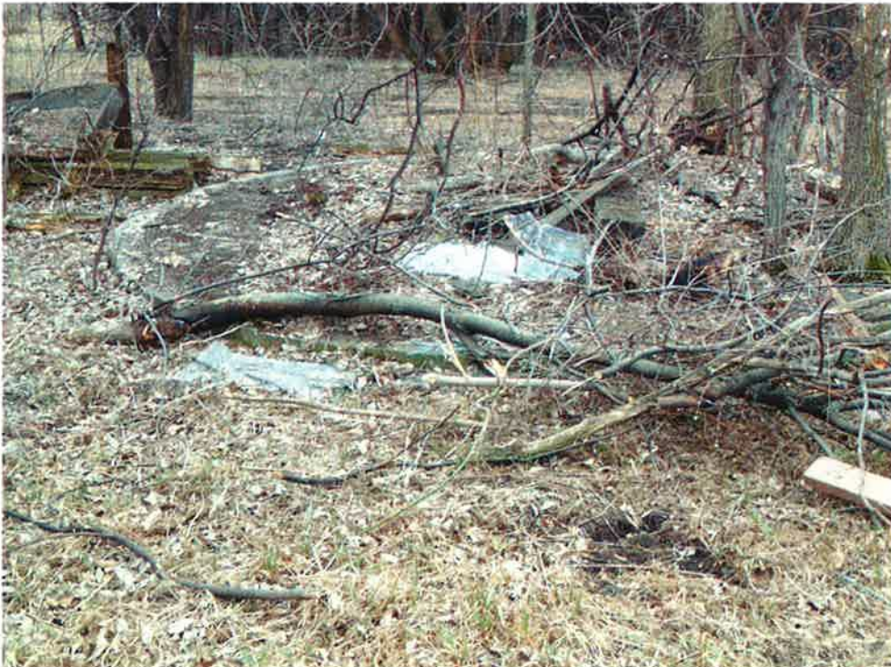
Figure 88. Feature 6, silo foundation, looking to the west.
