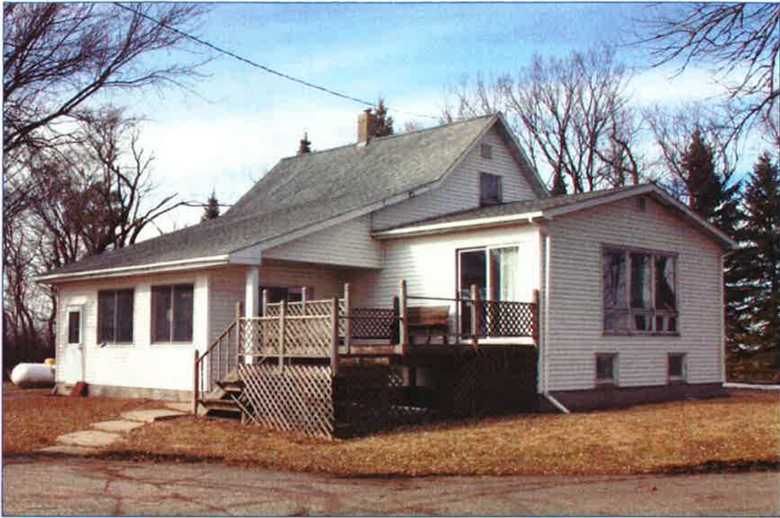
Figure 71. Southeast corner angle of Feature 1. View to the northwest.
