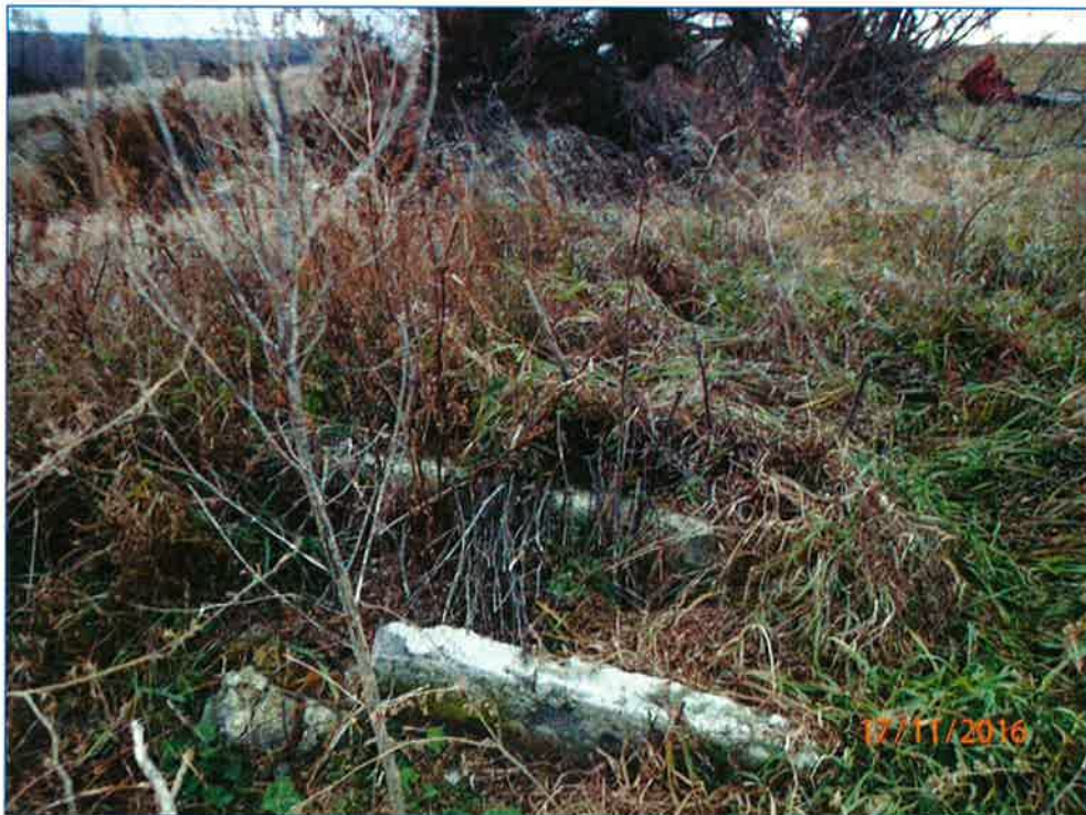
Figure 61. Feature 6: Fragmented foundation view to the west.
