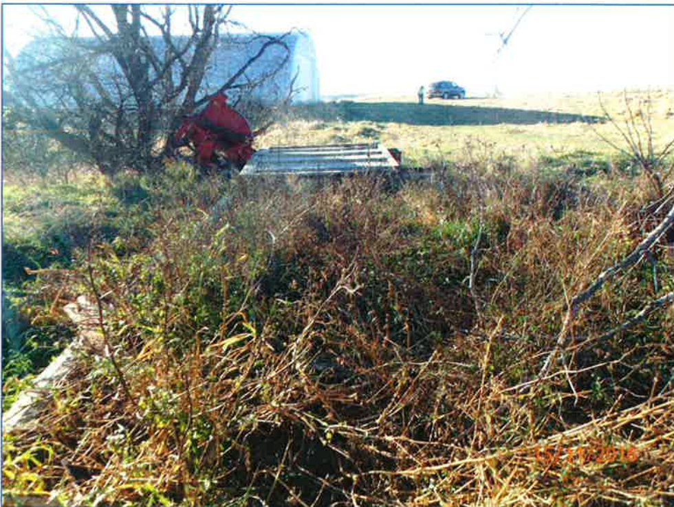
Figure 57. Feature 2: Foundation to the west.
