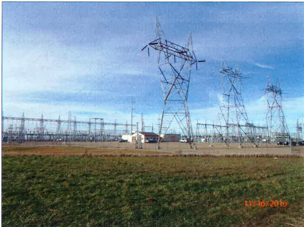
Figure 52. Site 21CP11 overview to the northwest.
