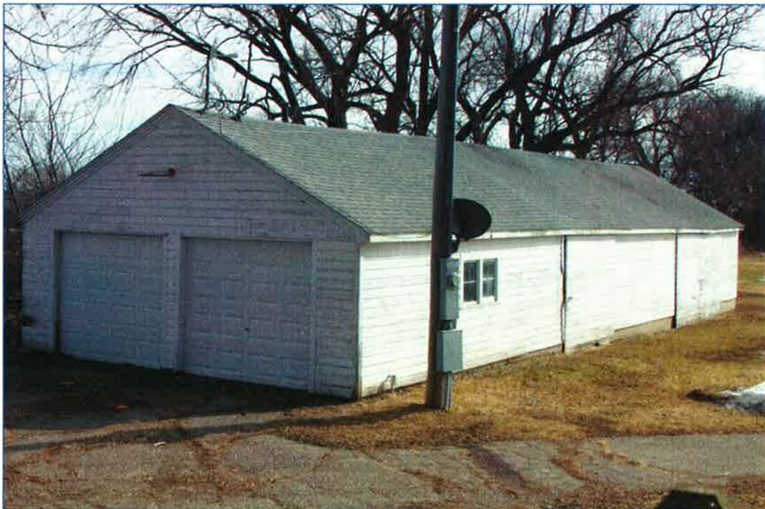
Figure 72. Northwest corner angle of Feature 2. View to the southeast.
