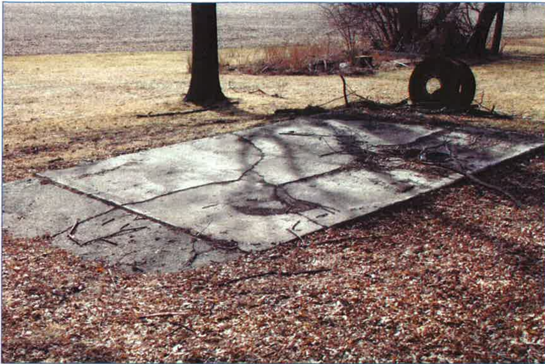
Figure 79. A modern concrete pad. View to the southwest.
