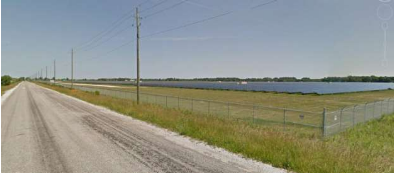
Figure 5: 80 Acre Solar Farm, Lambton County Ontario 54
