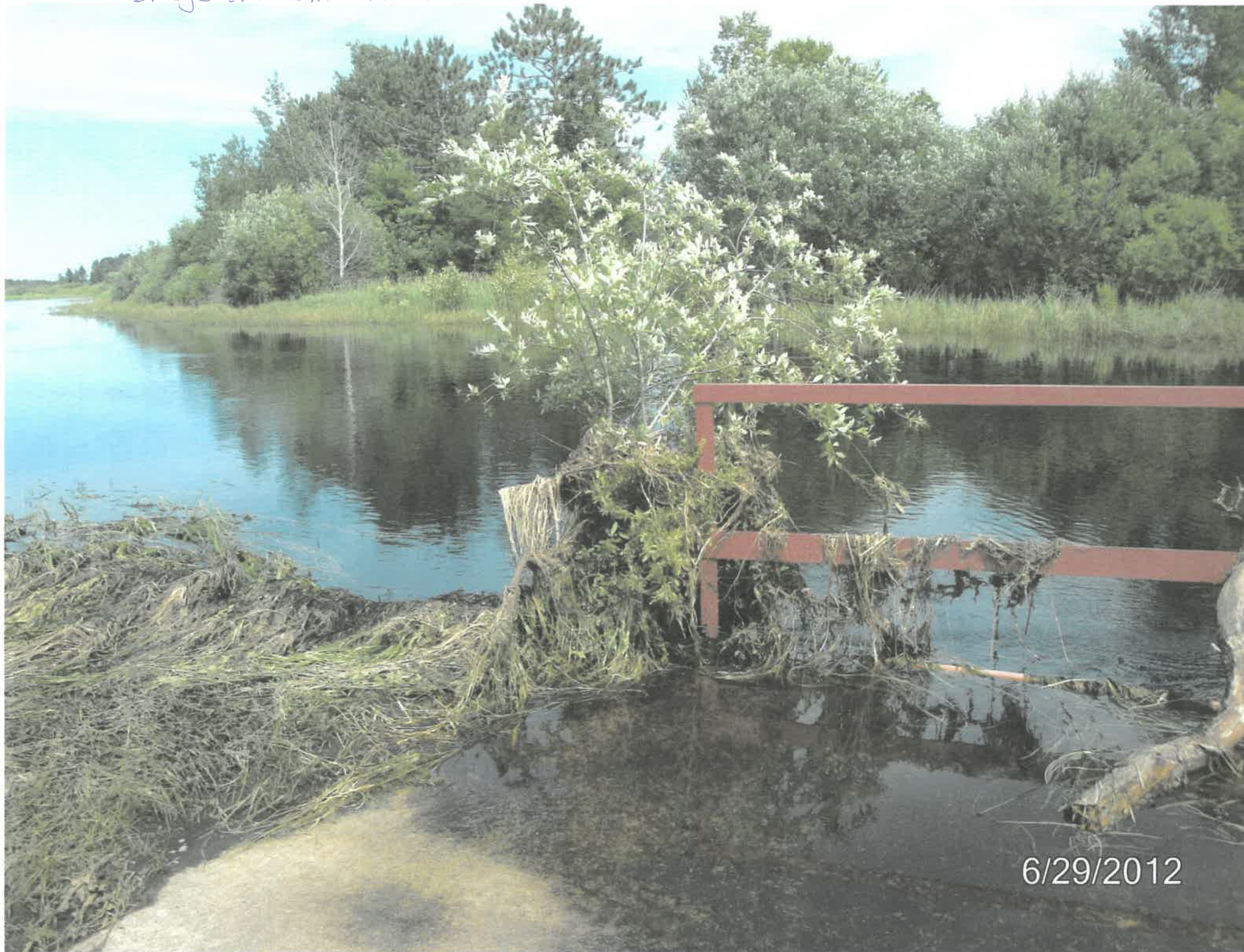
Bridge over Tannock River
