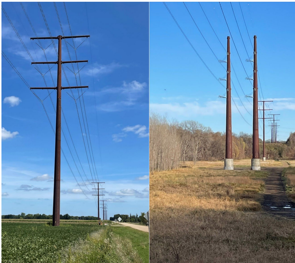
Typical Double Circuit Structures | Typical Dead-end Structures
