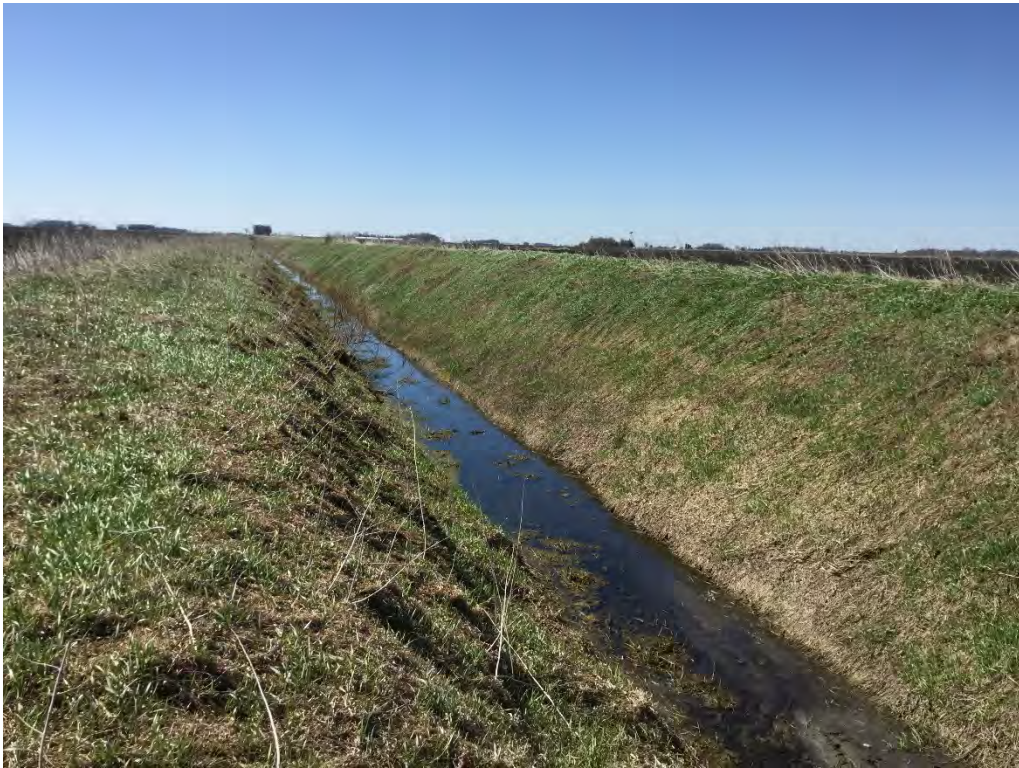
Photograph 5 (North): An overview of SA042.
