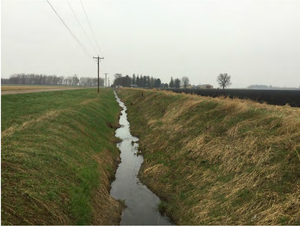
Photograph 1 (North): An overview of SA008.
