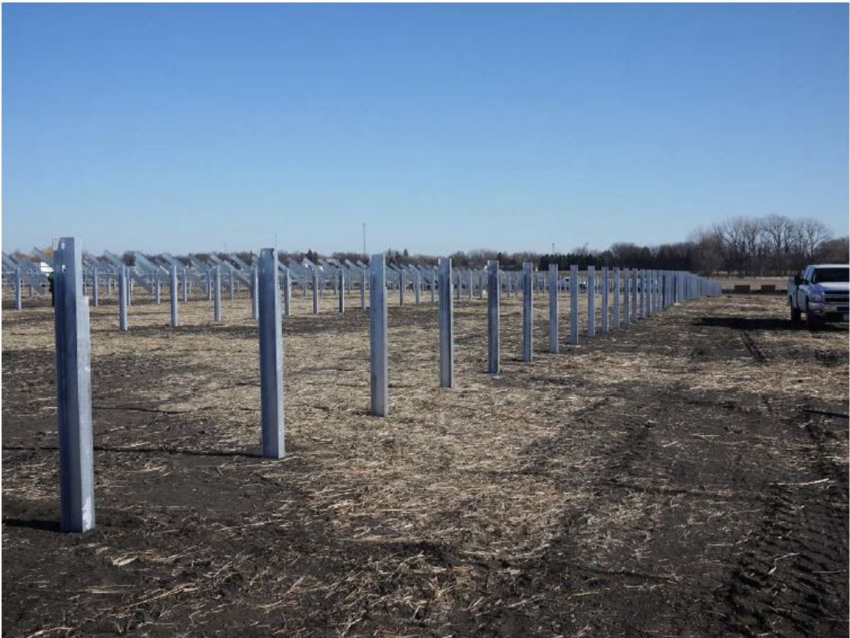
Diagram 6. Standard Steel Pier Foundations 42
