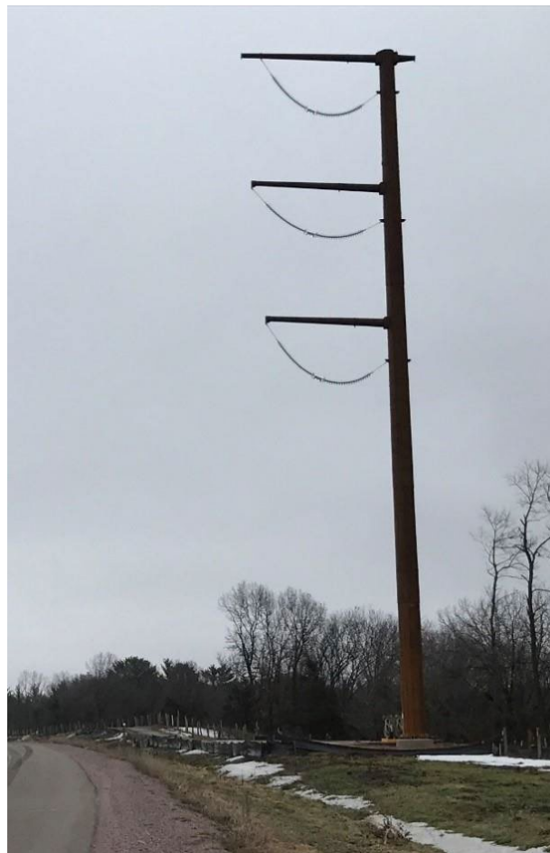
Diagram 12. Example: Single-Circuit Monopole 345 kV Structure 71
