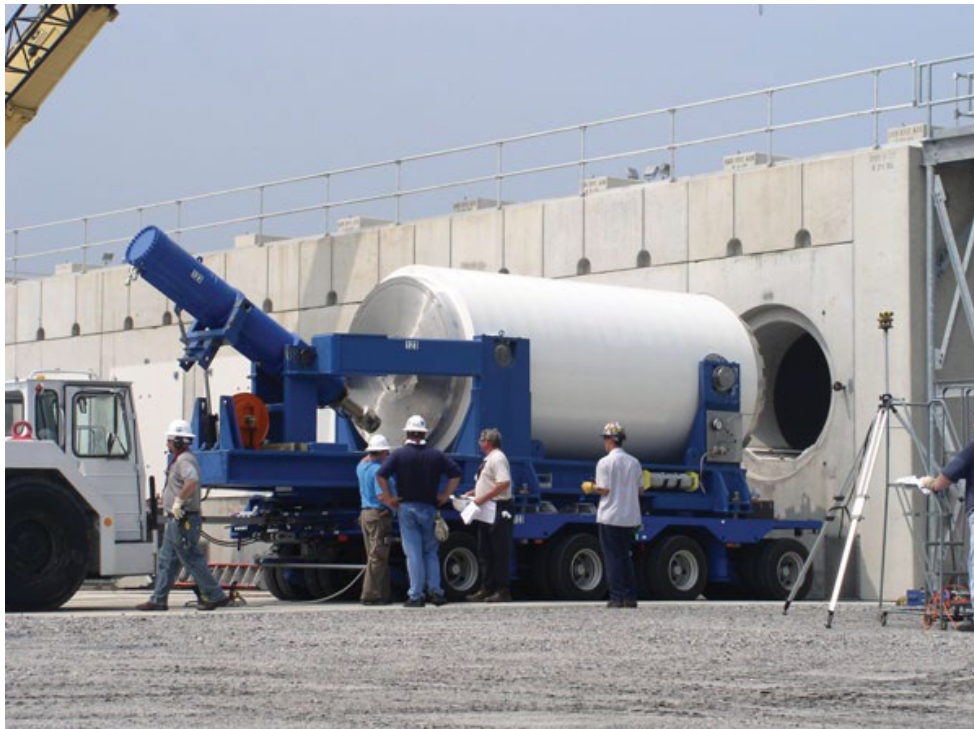
Figure 9. Canister Being Placed in Horizontal Concrete Storage Module
