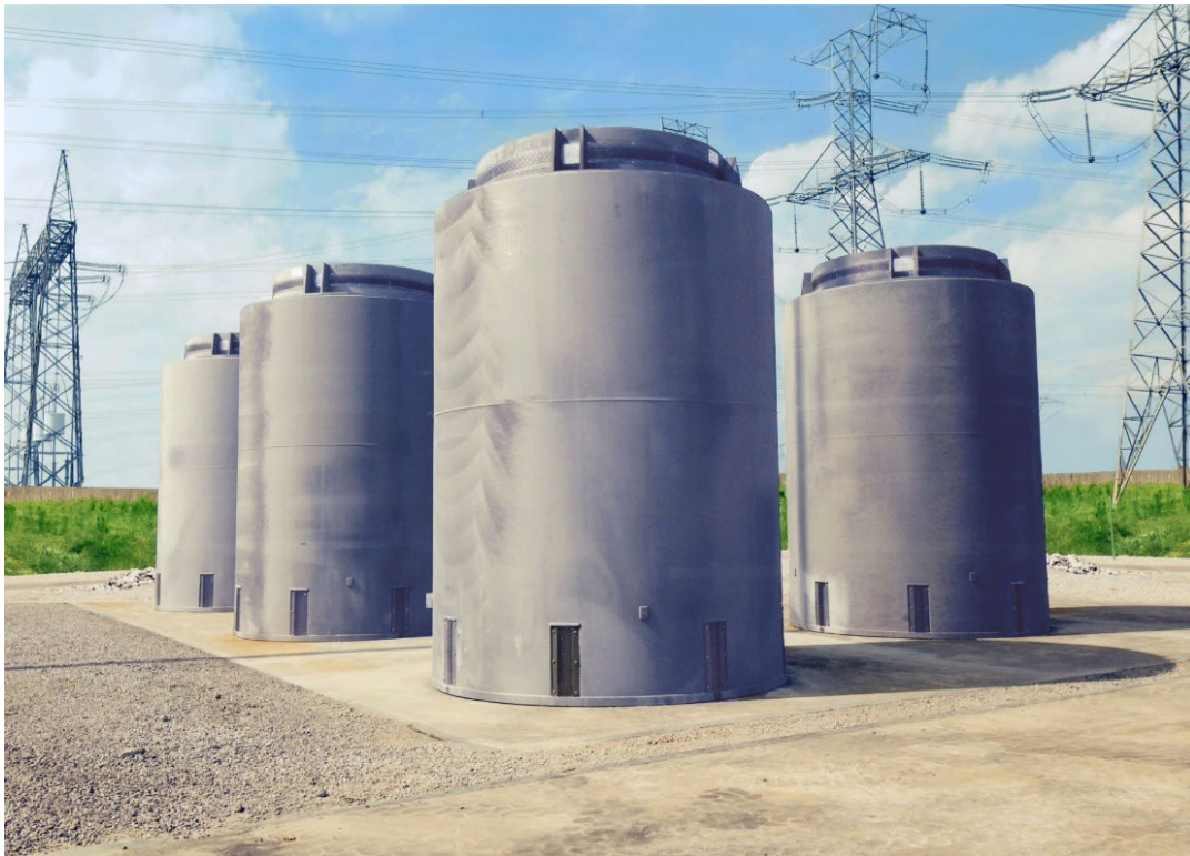
Figure 3. Vertical Canisters in Concrete Overpack
