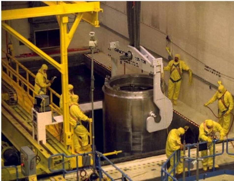
Figure 7. Canister and Temporary Metal Overpack Being Decontaminated
