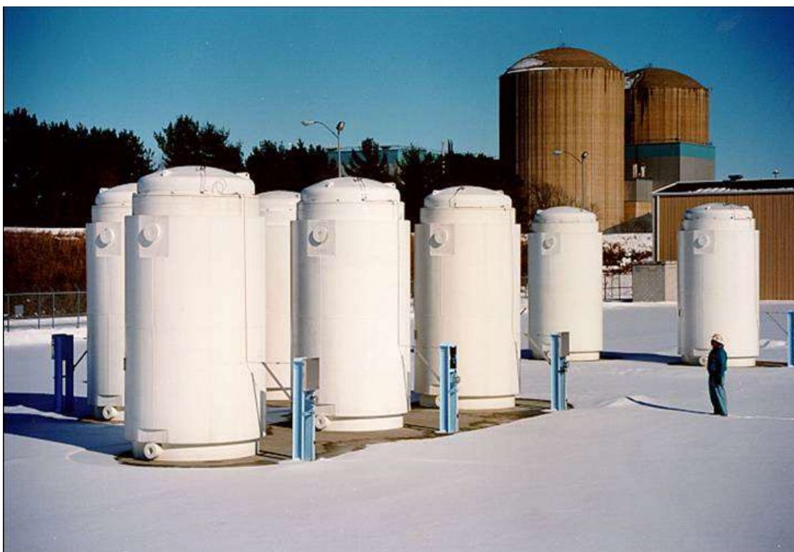
Figure 2. TN-40 Casks on ISFSI Pad
