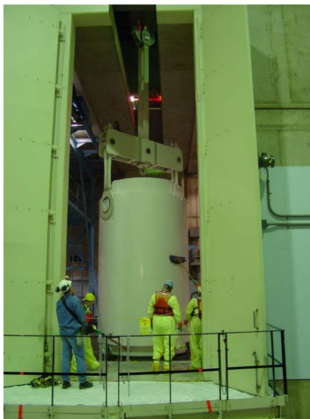
Figure 5. TN-40 Cask Removed from Spent Fuel Pool
