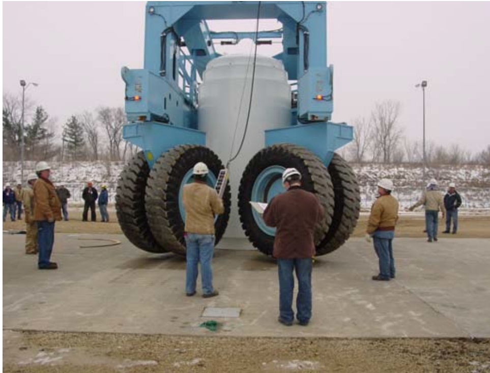
Figure 6. TN-40 Cask Placed on ISFSI Pad
