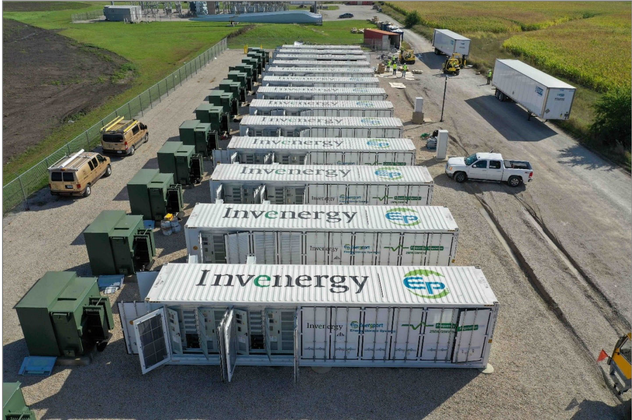
Image 5: Example of a BESS Containers
