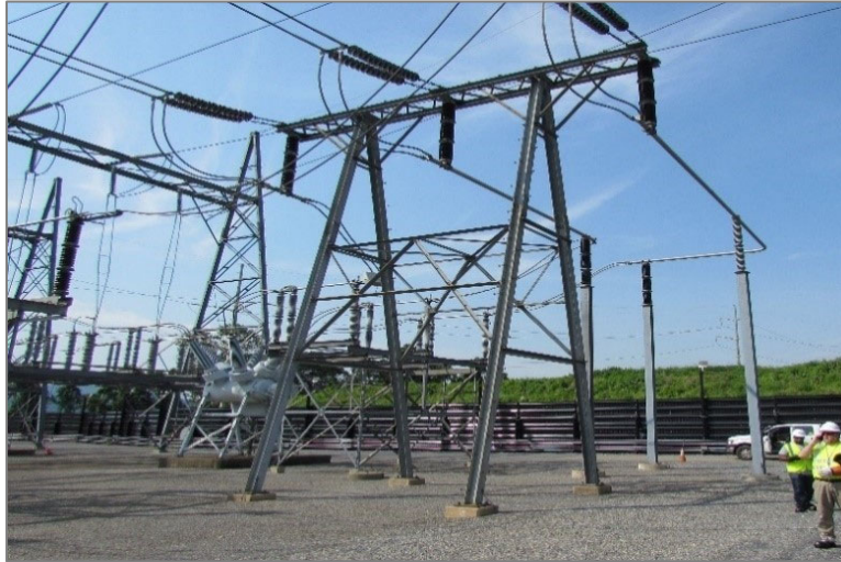
Image 3: Typical A-Frame Deadend Structure
