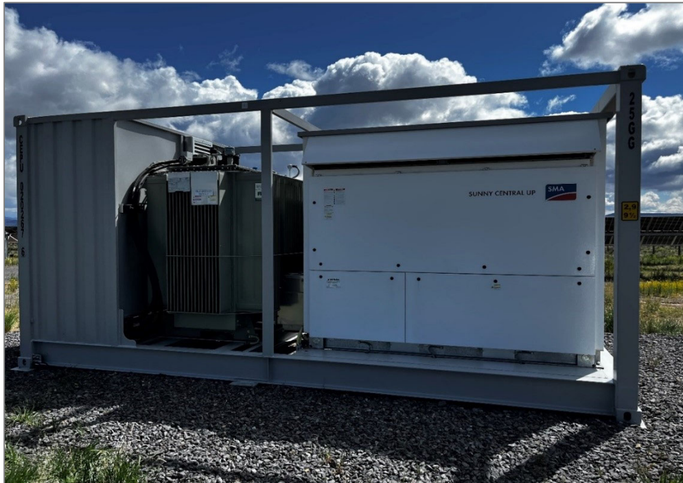
Image 7: Example of Inverter Skid (DC Cables Buried)
