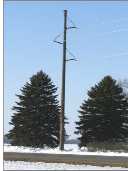
Image 4: Typical Overhead Transmission Line Structure
