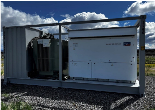
Figure 4: Typical Inverter Skid
