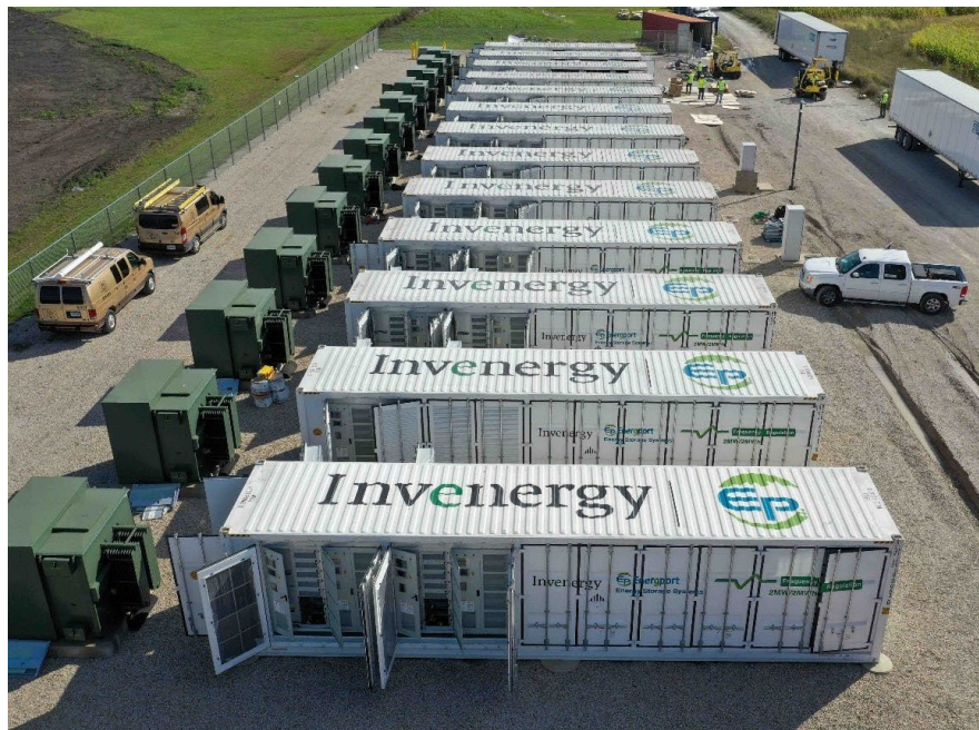
Figure 3: Typical BESS Container Configuration
