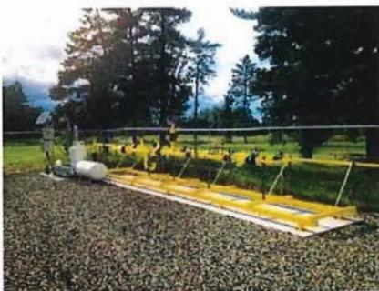
This Northwest Gas equipment is used for gas pressure reduction and odorization.
