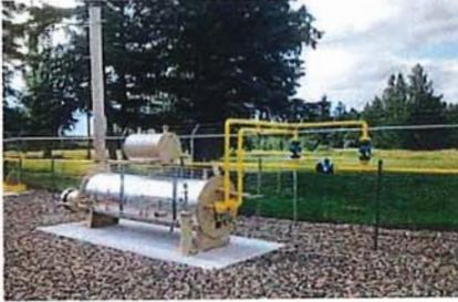
This Northwest Gas photo shows a gas-fired waterbath line heater installed to heat the system gas.
