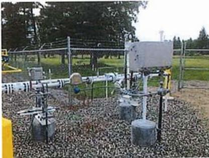
A Coriolis meter installed in the high-pressure piping coming from the transmission line measures incoming gas.
