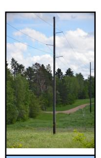
Typical 115 kV Transmission Structure
