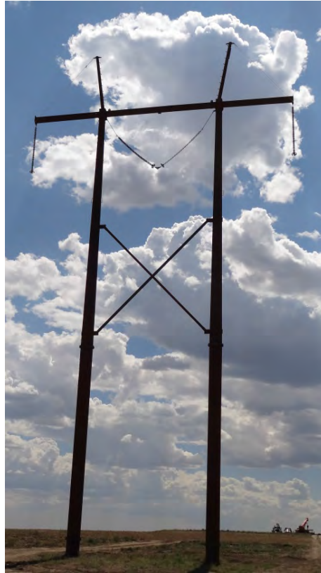
345 kV Steel Single-Circuit H- Frame Structure
