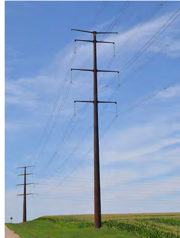
345 kV/345 kV Steel Double-Circuit Monopole Structure 10
