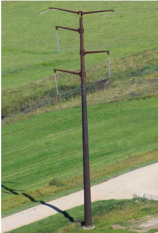
345 kV Steel Single-Circuit Monopole Structure
