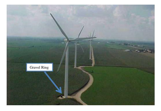
**Figure 6: Gravel Rings and Access Roads**
