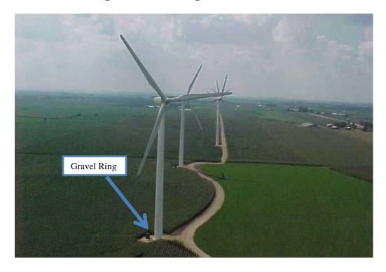
Figure 6: Gravel Rings and Access Roads
