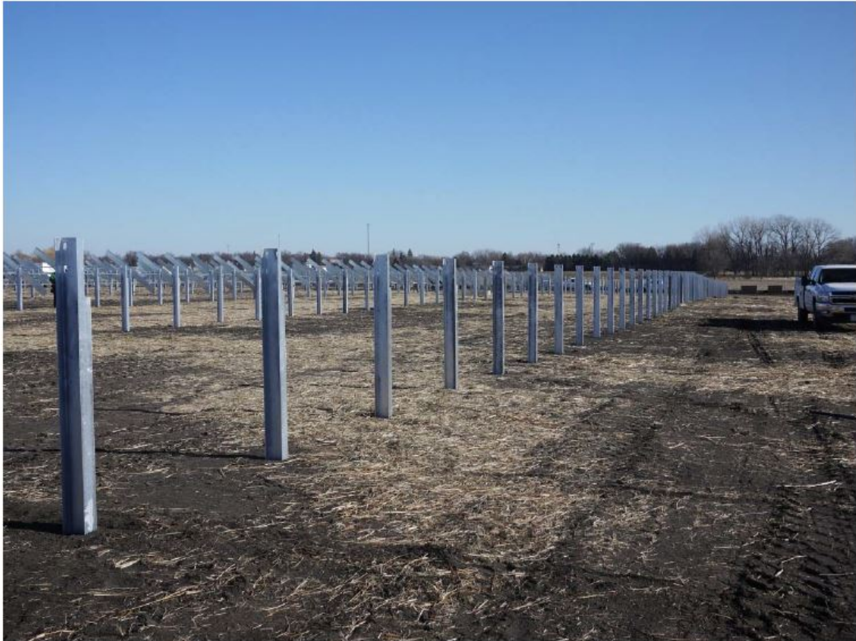
Image 5: Standard Steel Pier Foundations
