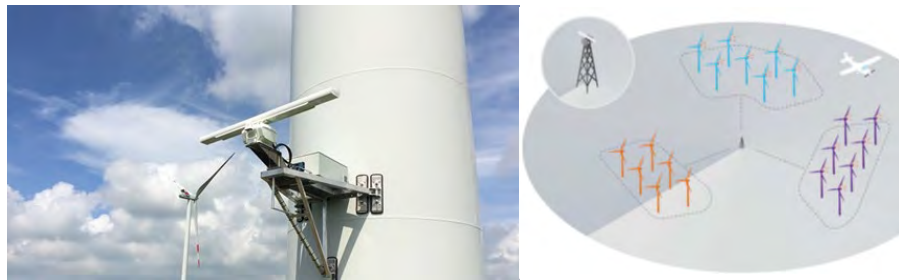
Diagram 22. Aircraft Detection Lighting System 222
