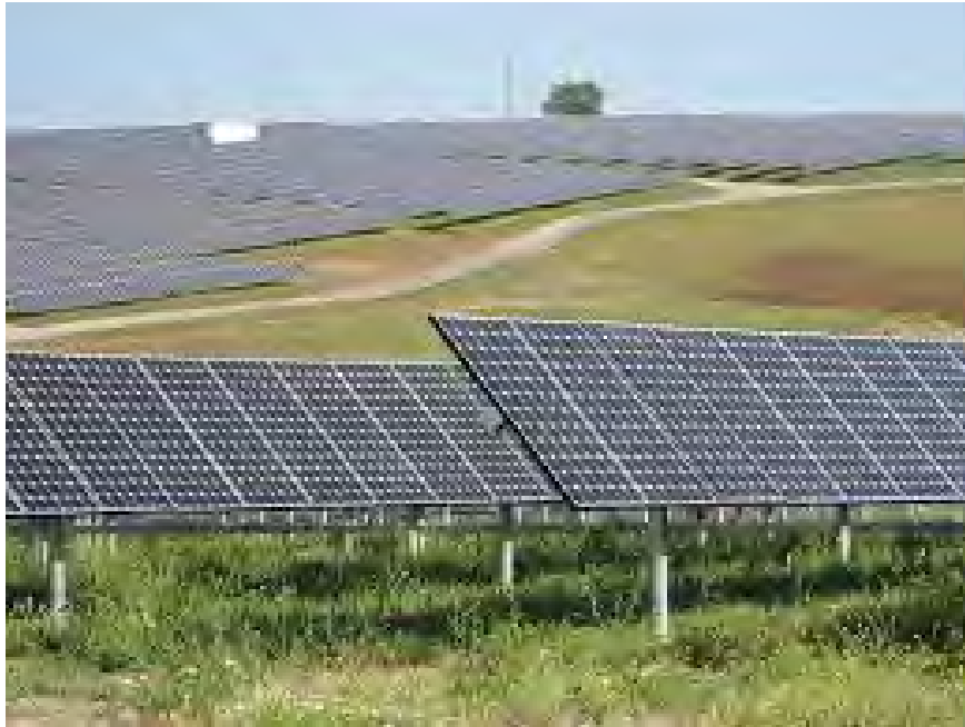
Diagram 5. Arrays Mounted onto Tracking Rack System 34
