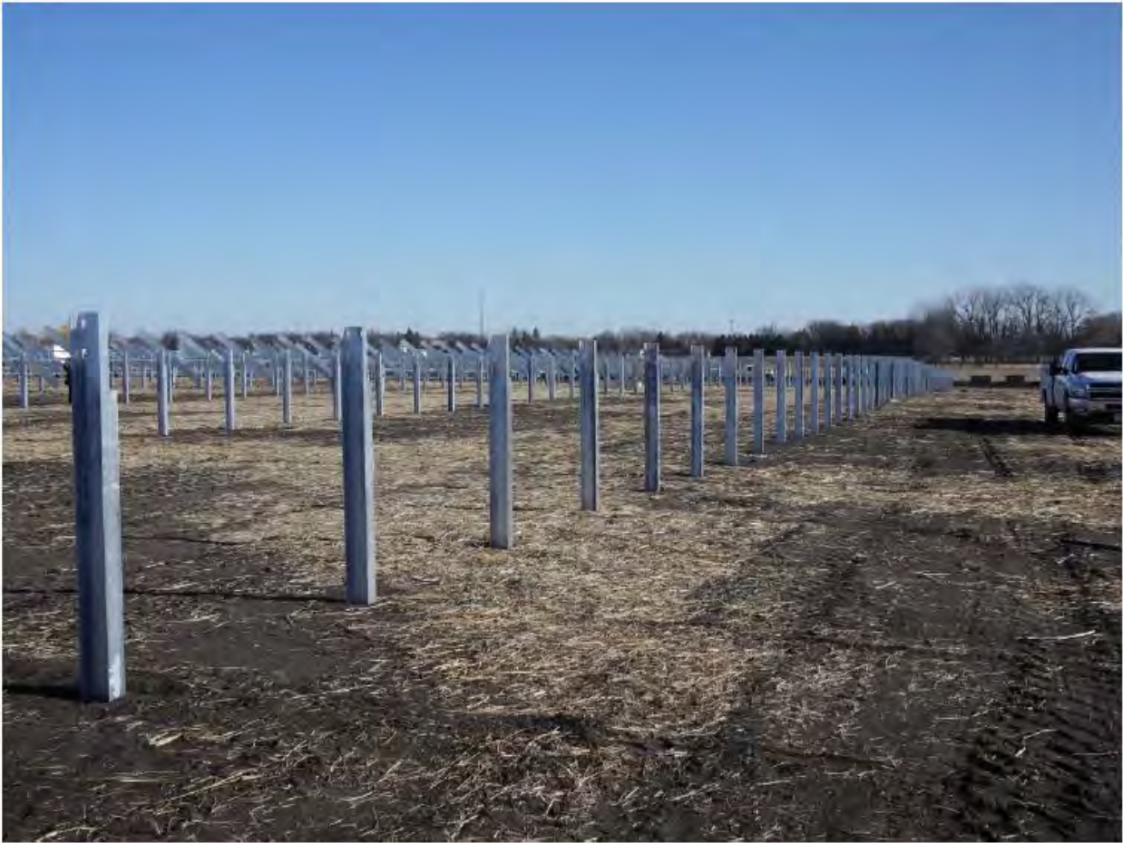
Diagram 7. Standard Steel Pier Foundations 36
